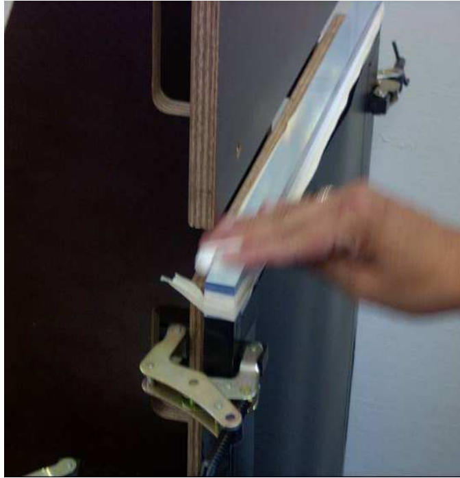
Figure 17: Cleaning the surfaces
